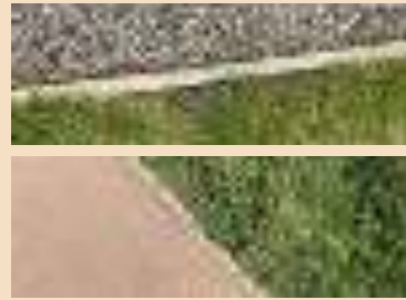
Timber edge (above) Concrete 50mm kerb (below)
